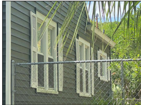
Figure 2: Example of non-historic windows installed with traditional amount of reveal, 2709 Burlington Ave. N.
