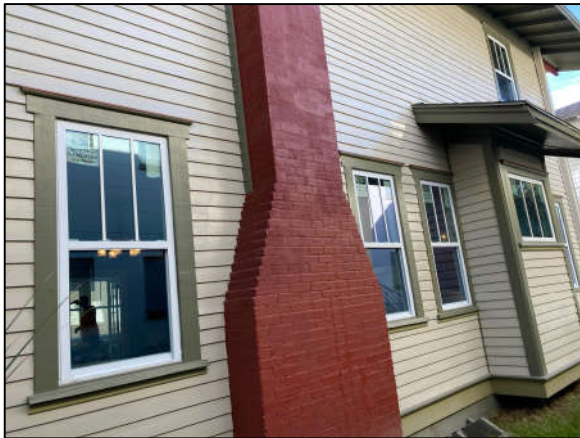
Figure 1: Replacement windows after installation at primary residence, 812 8 th Ave. S., 2020
